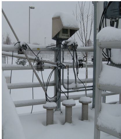
The IQ SensorNet 2020 XT terminal mounted tank side provides continuous process monitoring and control - even in harsh conditions.
